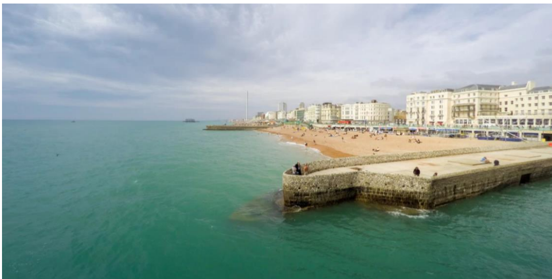
Figure 6-1: Breakwater at Brighton Seafront
